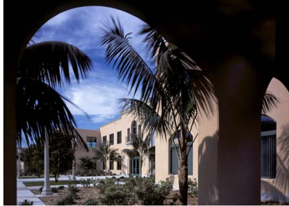
Office Building at NTC
